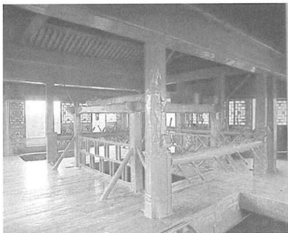
Fig. 4. Five handspike windlasses for the lifting apparatus located in the backstage of the Fortune Stage of the Pleasant Sound Pavilion. Photo from Yú Zhuōyún 于倬云, Zìjìn Chéng Gōngdiàn 紫禁城宫殿, p. 166, plate 184.
