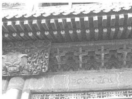
Fig. 5 a. The bracketing system in the east side of the three-tiered stage the Pleasant Sound Pavilion. Photo taken by Sasiporn Petcharapiruch on November 11, 2004.
